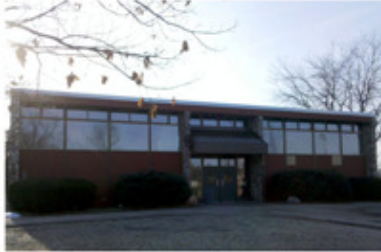
View of the new Philippine Center at the Zablocki Park Pavilion
