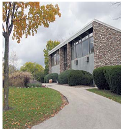
Front View from Parking
