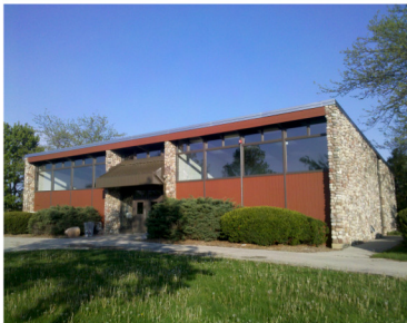
View of the Zablocki Pavilion/ Philippine Center showing new canopy at the main entry
